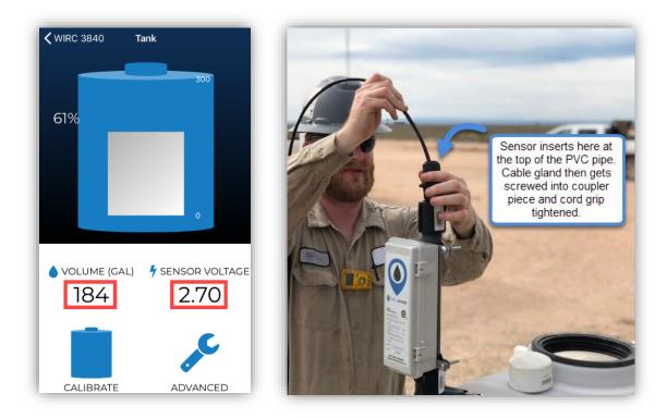
Now you can tighten your cord grip on top of the WIRC assembly. Be certain the cable is snug on the sensor wire but not too tight that it can crush or kink the reference tube. Then be sure to place the chemical tank cap back in place.
