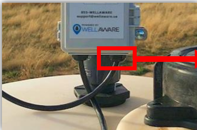
Tighten cord grip to prevent sensor cable movement.
